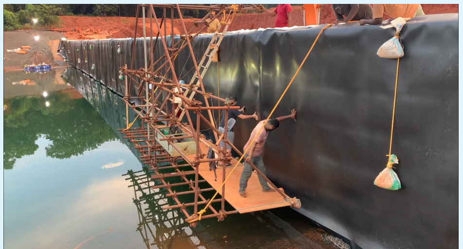
The walls of the test Lake have now been raised to 8.3 meters height and waterproofed, ready to hold the rain water harvest from the upcoming monsoon.
